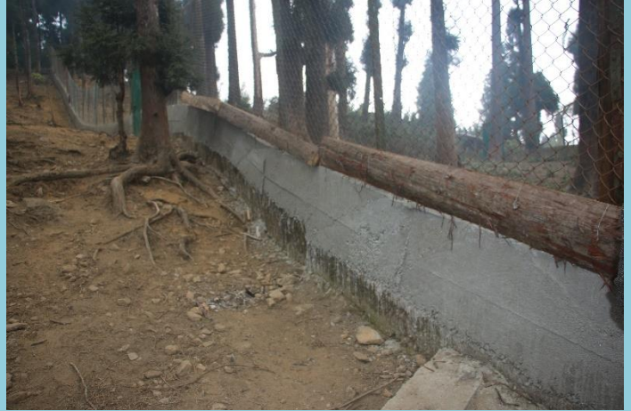
Bamboo fencing and partial concreting of the bamboo fences in the herbivore enclosures at the conservation breeding centre for herbivores and pheasants at Dowhill, Kurseong.
