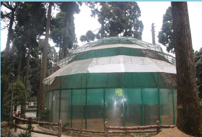
Modified roofing for proper drainage in the circular pheasantry and nesting area at the conservation breeding centre for herbivores and pheasants at Dowhill, Kurseong.
